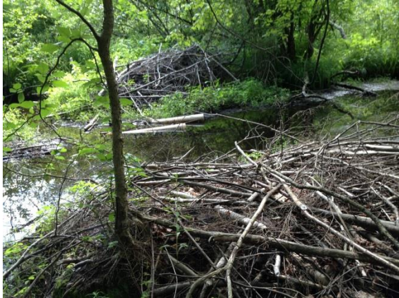
View of inactive breached beaver dam at Area 20.
