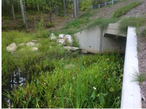
View of Upstream side of culvert at Area 1.
