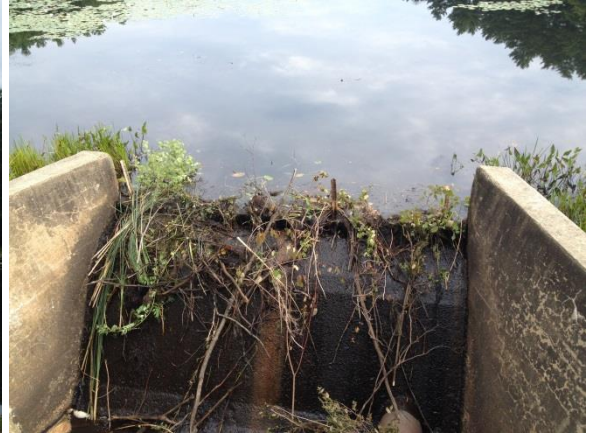
View of the Stump Pond spillway.
