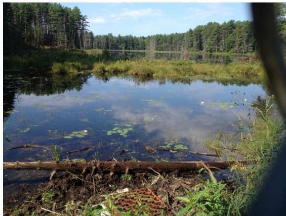
View of the Greens Pond drop inlet from Greens Pond Rd.
