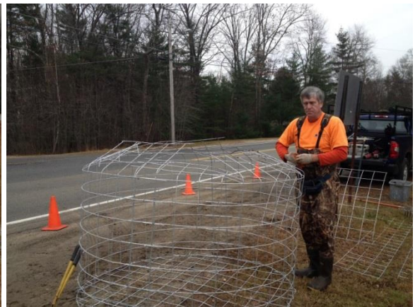
Six gauge steel panels are used to construct protective panels. The panels are cut, rolled, and bent to form an approximate 5.75 foot wide and 3.75 foot wide protective fence to surround the inlet of an HDPE pipe.
