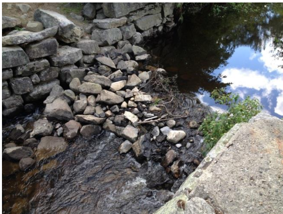
View of old granite bridge known as "Twin Bridges."
