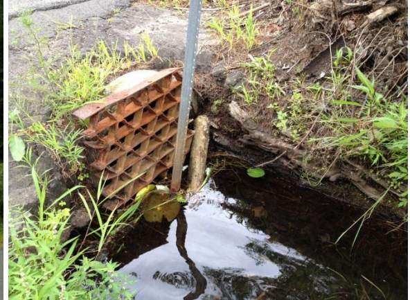
View of road culvert requiring period maintenance.
