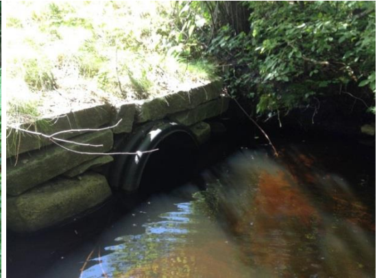
View of Area 2 culvert outlet.
