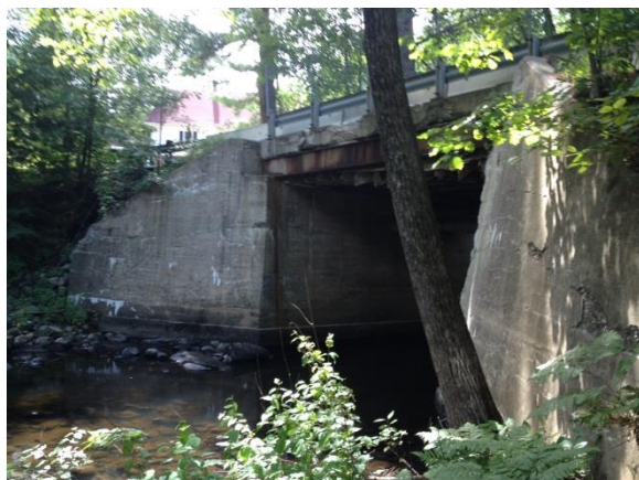
View of McGraw Bridge Road.
