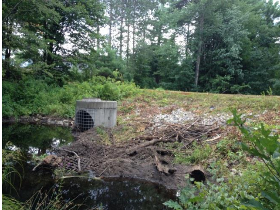
View of sewer line area looking towards Mayflower Road.
