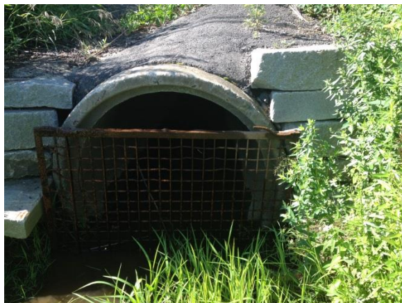
View of Lyons Road culvert and grate.
