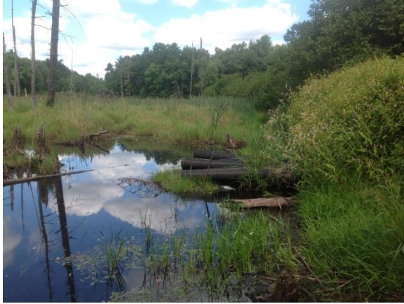
View of culverts installed on Summitt Road to prevent plugging by beaver. These limit flow and wildlife passage.
