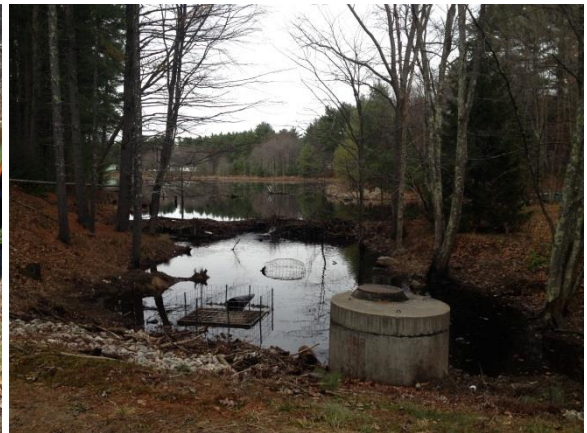
View of installed devices. The Flexible Pond Leveler in the main beaver dam is submerged.
