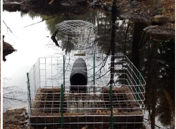
View of protective fence installed at the inlet to Meadowwoods Dam.
