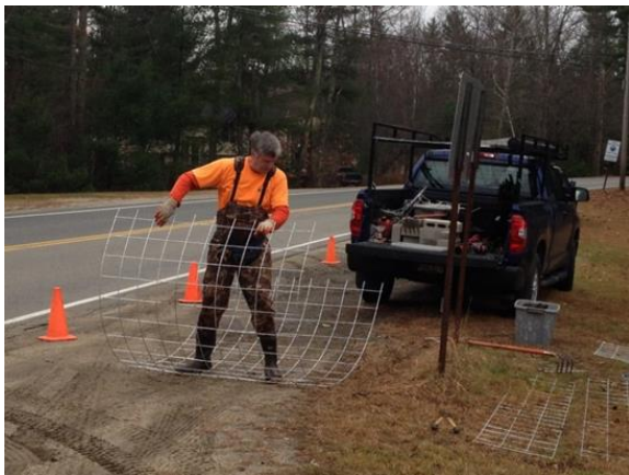
Six gauge steel panels are used to construct protective panels. The panels are cut, rolled, and bent to form an approximate 5.75 foot wide and 3.75 foot wide protective fence to surround the inlet of an HDPE pipe.
