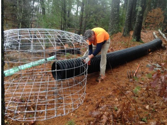
View of construction of Flexible Pond Leveler.
