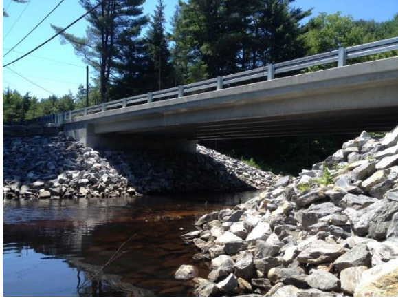
View of Wire Road Bridge.
