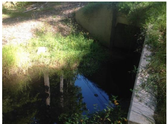
View of downstream side of Area 1 culvert.
