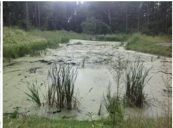
Overall view of detention pond.
