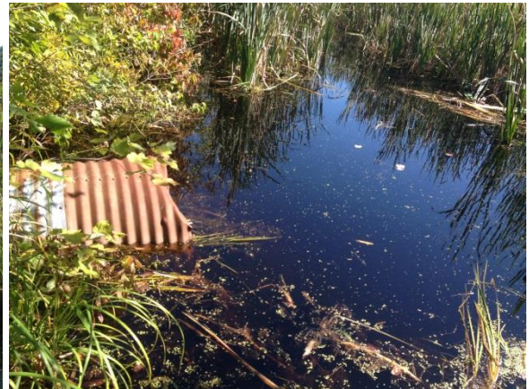
View of culvert at Area 24.
