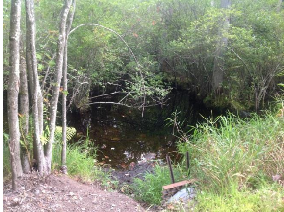
View of Area 14 culvert and protective grate.
