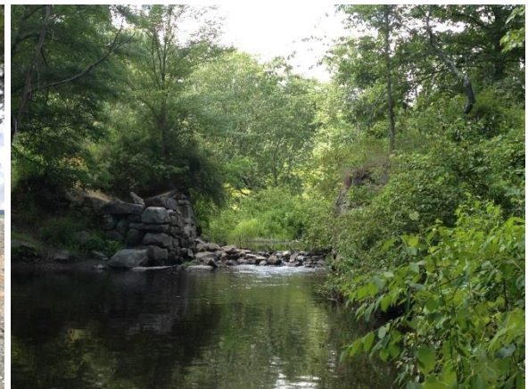
View looking upstream at Twin Bridges.
