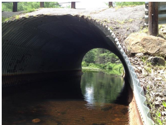
View of Area 3 looking upstream at the culvert.
