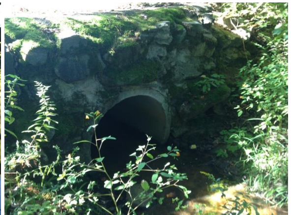
View of Merrymeeting Road culvert.
