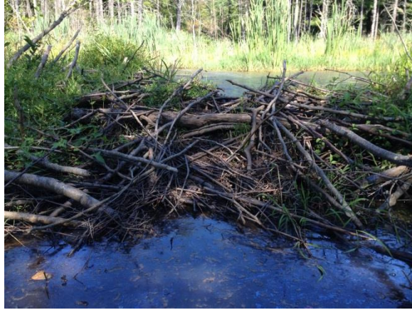
View of primary beaver dam in Area 15.
